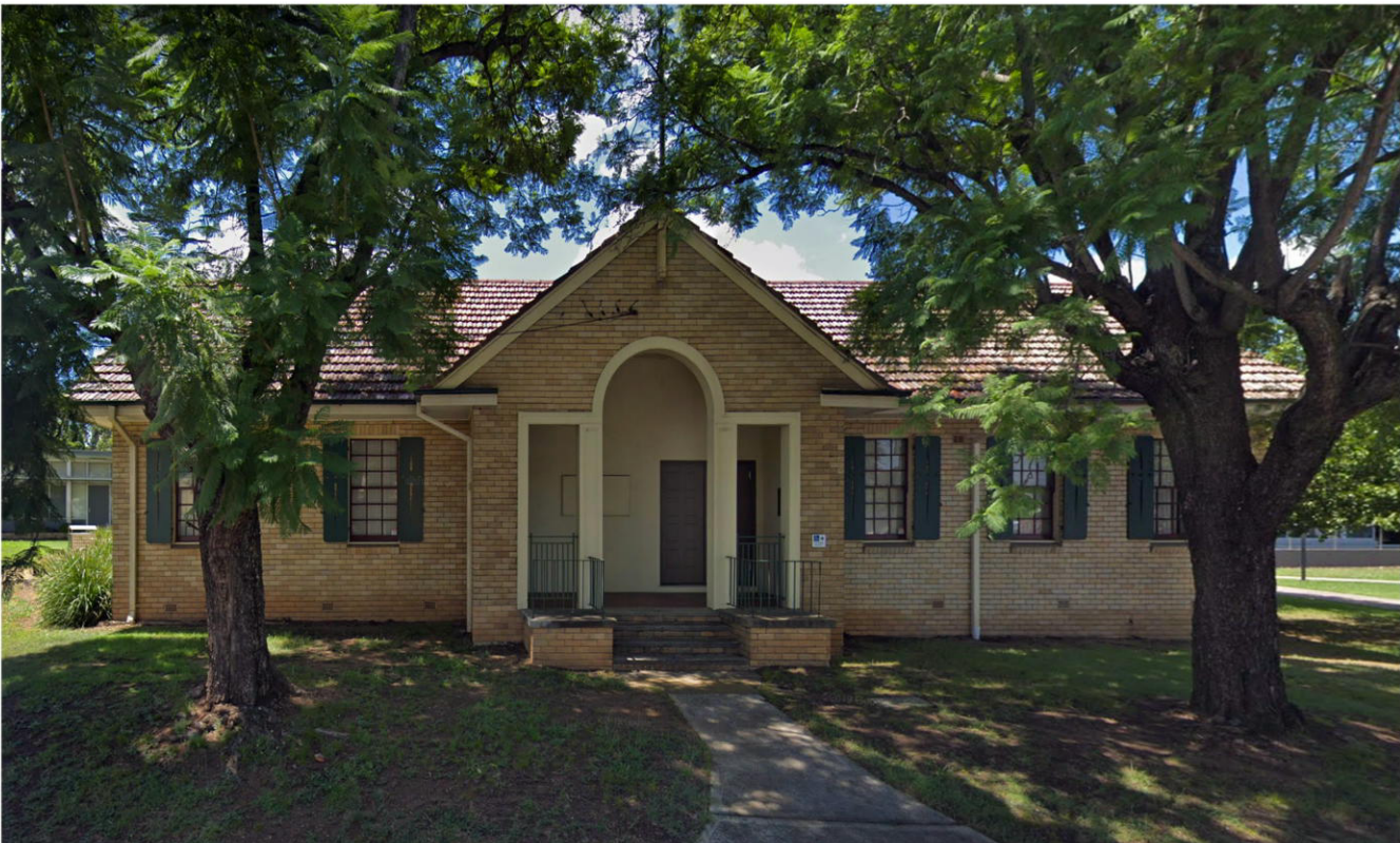
Former Council Chambers 3 Mamre Road, St Marys Constructed 1933, light coloured brickwork, timber framed windows with vertical proportions, external shutters
