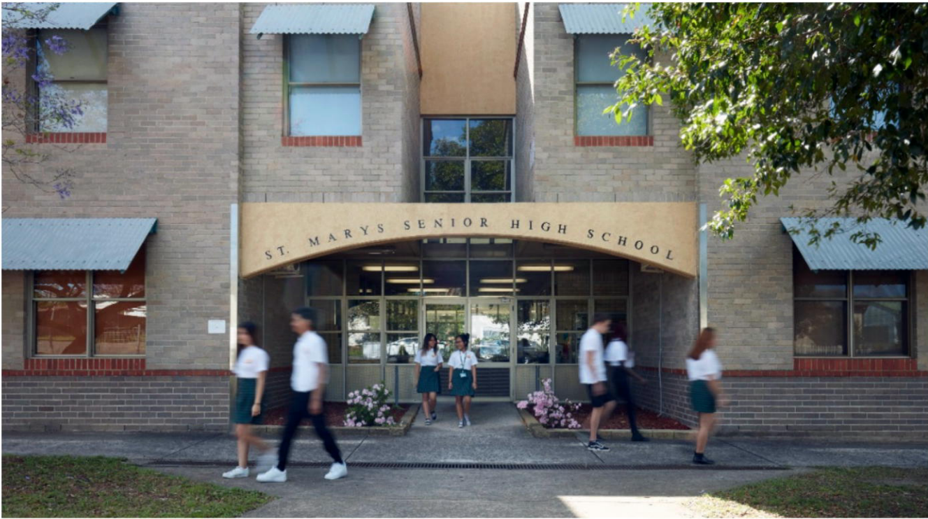
St Marys Senior High School 6-48 Kalang Avenue, St Marys light coloured face brickwork with darker base course, aluminium framed windows with vertical proportions, lightweight metal sun hoods
